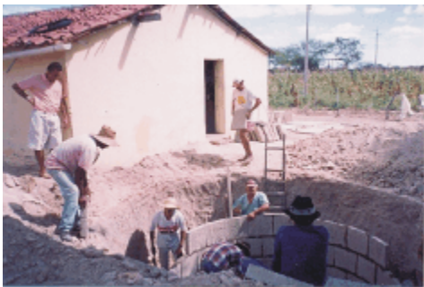
Figure 4.8. Construction of a Cistern
